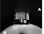
Step 2 Insert the calmed inlet elbow in to the smaller of the two holes.
